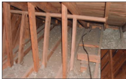
Top: The "insulation" in a home during an initial audit. Under the weatherization assistance program (bottom), crews installed an R30 blanket – which should lower the home's energy usage.
